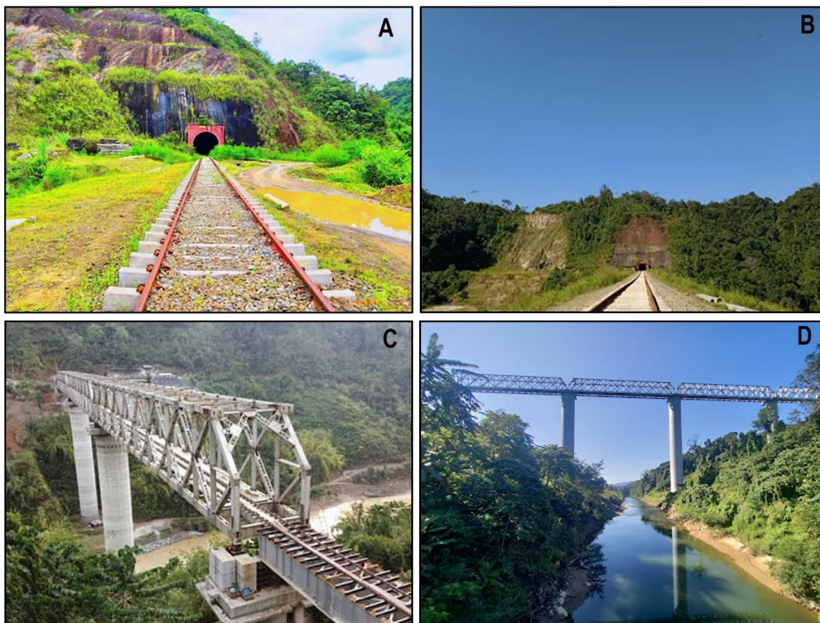
Figure 6. Different railway tunnels (A-B) and bridges (C-D) in Manipur railway
