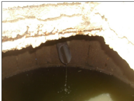
Figure 3. Exterior of a pit showing the evacuation pipe for specifically hospital effluents
