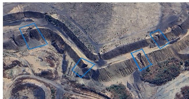
Figure 2. Subsurface flow channels contribute to the erosion of slope material, compromise the stability of slope margins, and can ultimately lead to slope failures
