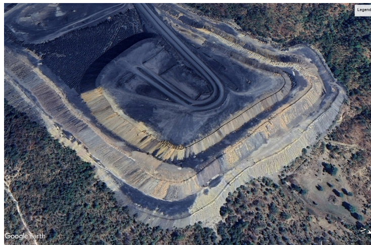
Figure 1. IZUMA dump slope
