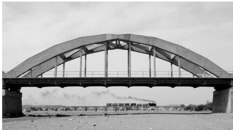
Figure 4. Massawa Bridge (1938) with the characteristic hinge in the arc to reduce thermal stress
