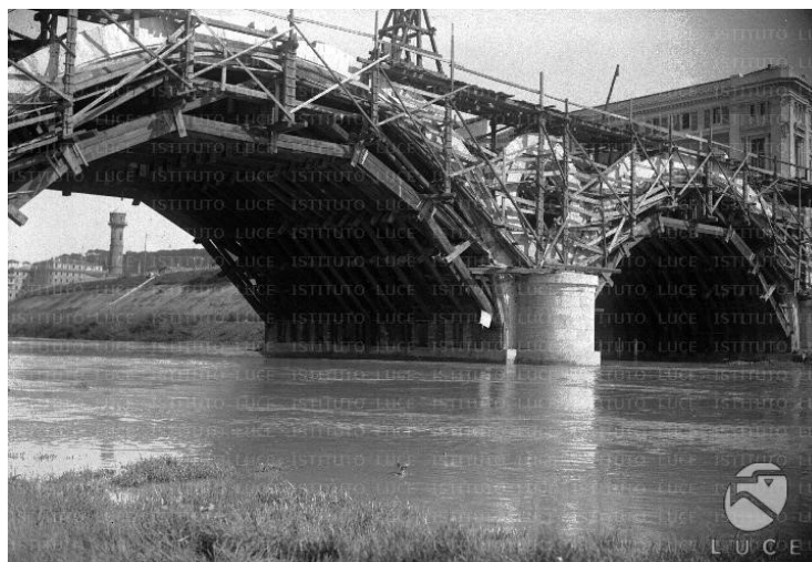
Figure 2. Construction of the Eugenio Miozzi’s Liberty Bridge – Venetian Lagoon - Italy (1931)
