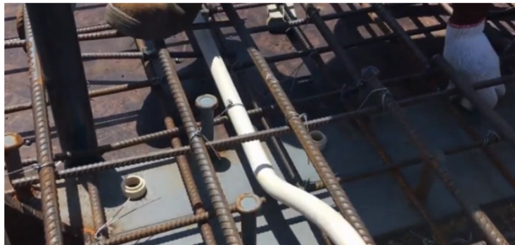
Figure 7. Angle welding on steel element
