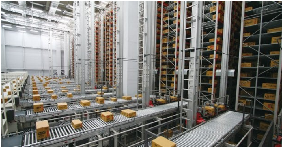
Figure 5. AS/RS in an automated warehouse [13]
